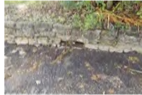
1426 Retaining Wall near Public Works Building
