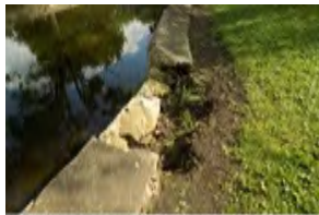
Allen's Creek Rip-Rap at East L
