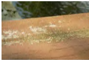
507 Allen's Creek Footbridge
