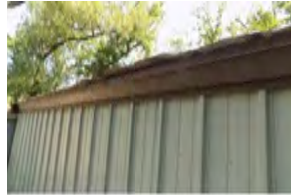
1425 Department of Public Works Building
