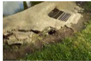
Allen's Creek Rip-Rap at East L
