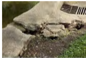
Allen's Creek Rip-Rap at East L
