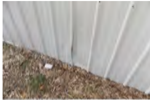
1419 Department of Public Works Building
