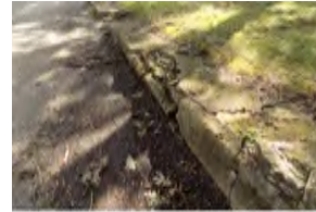
1427 Retaining Wall near Public Works Building
