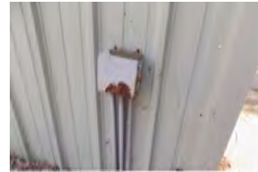
1422 Department of Public Works Building
