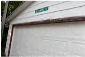
1418 Department of Public Works Building
