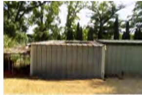
1420 Department of Public Works Building
