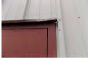
1424 Department of Public Works Building
